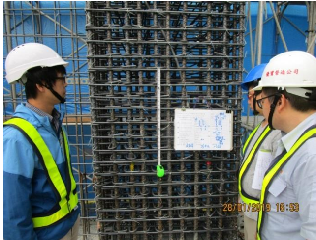
◎ Step.5 柱筋綁紮施工抽查驗
