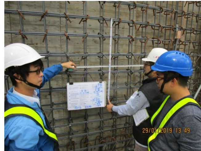
◎ Step.6 牆筋綁紮施工抽查驗
