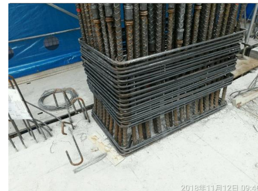
柱偏位任意偏折柱主筋
